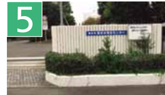
5 Kanazawa Water Reclamation Center*
